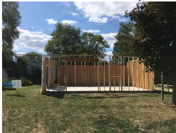
8-24-19 All four walls up
