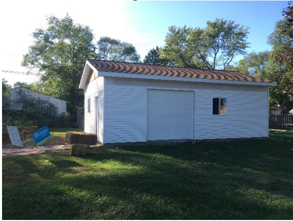
9-26-19 Garage door installed
