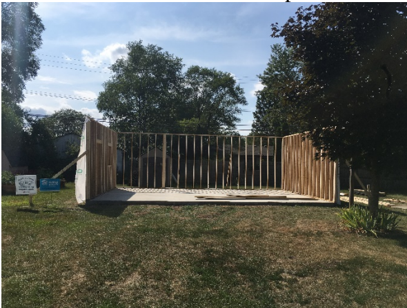
8-17-19 First walls up
