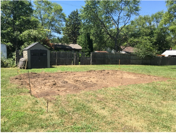
7-20-19 Foundataion slab prep
