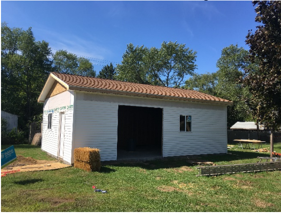
9-19-19 Roof on & siding started
