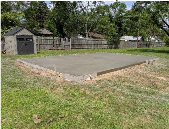
7-26-19 Foundation slab poured
