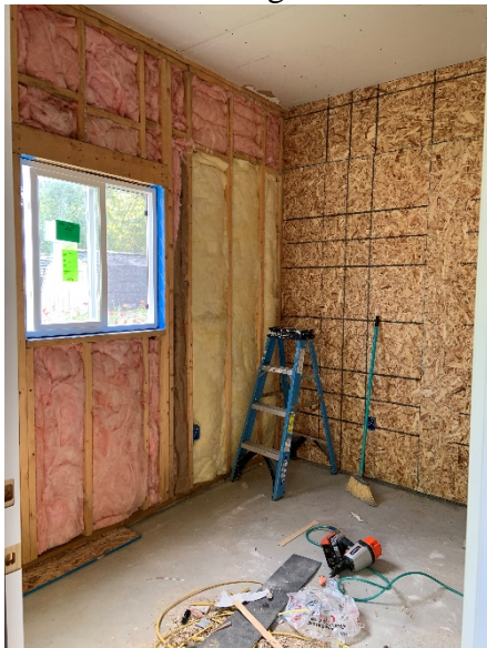
10-10-19 Insulating the office and hanging sheeting on the walls
