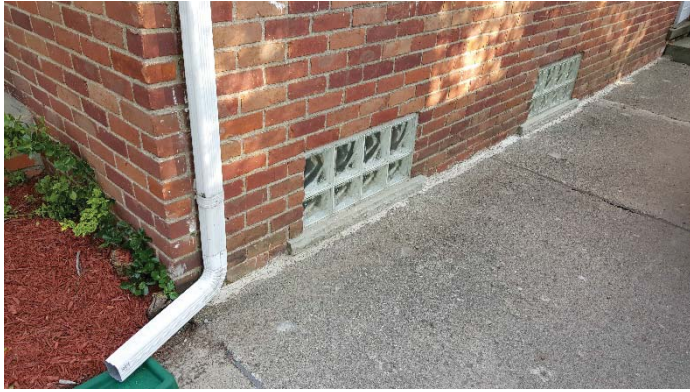
Foundation Caulk, Downspout Extension/Splash Block
