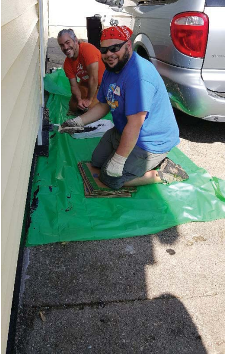
Painting Foundation Block
